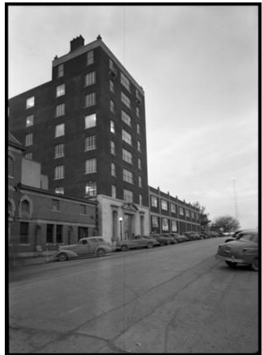
About 1930—the Steck Building was built in 1928 immediately adjacent to the Congregational church. After much discussion and several diagrams, it was determined that the front of the church was on W. 9th St.
