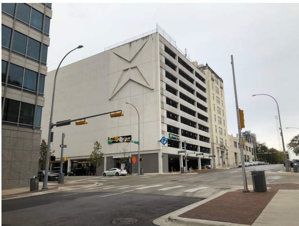
11/11/18 The intersection of 9th and Colorado, SW corner, where the original church building was located. Note again the entrance to what was the Steck Building
